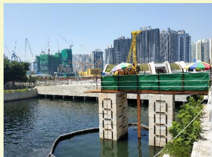
Pre-drilling works for vehicular bridges across Kai Tak River
