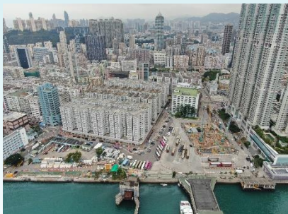
Construction of Access shaft & cut-and-cover tunnel at Ma Tau Kok
