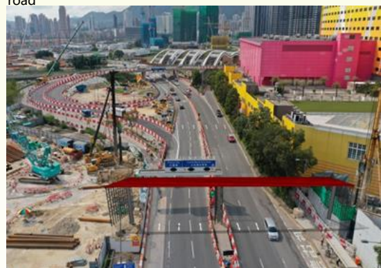
Photomontage of temporary falsework for construction of Kai Fuk Road Footbridge
