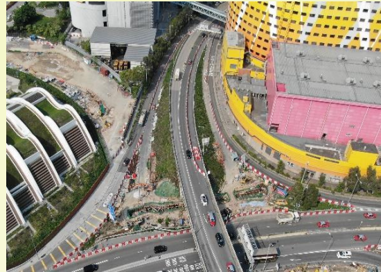
Temporary traffic arrangement for Kai Cheung Road U-Turn slip road
