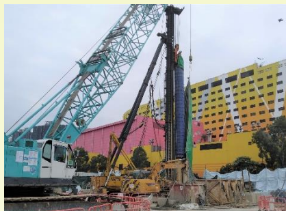
Piling works for Kai Fuk Road footbridge
