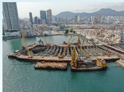
Construction of stage 1 underwater tunnel at Kowloon Bay
