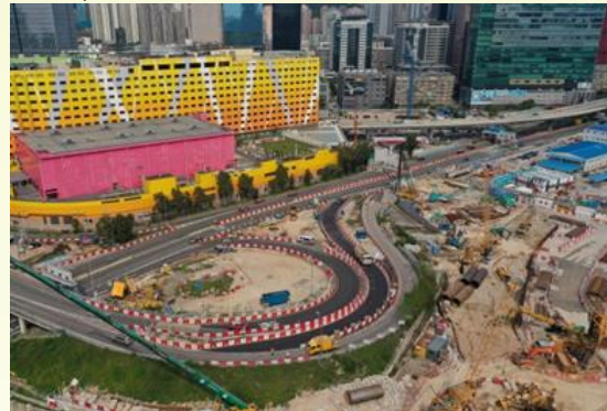
Temporary traffic arrangement for Kai Cheung Road loop road
