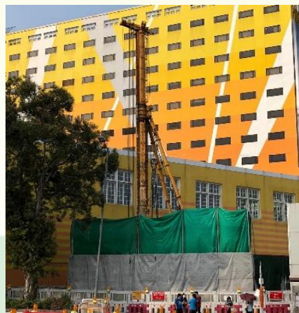
Erection of noise barrier at construction site
