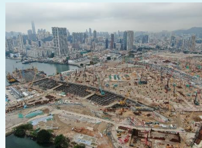
Construction of cut-and-cover tunnel, depressed road and underpass at Kai Tak
